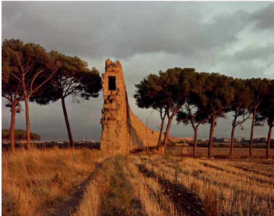
A view of the water channel of the Claudian Aqueduct and the Anio Novus Aqueduct piggybacked on top, near Cinecitta, Rome, December 1990
